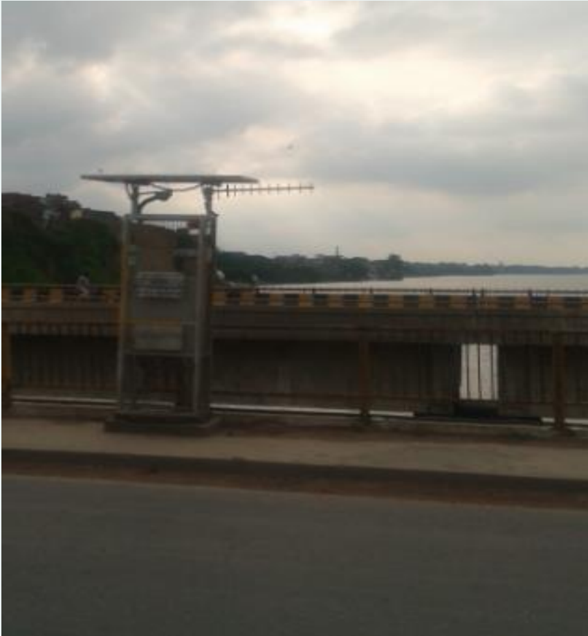
Jajmau Bridge Kanpur-Fixed
